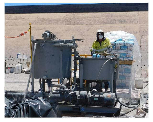
All the start and stop operations of the three main components (High shear mixer, agitator and grout pump) are managed by the control panel. Two valves open and close accordingly allowing the mixing of the product and its passage to the agitator tank. Another valve controls the flow of product into the cavity pump for delivery to site.
